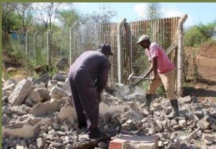
Demolition of the old gate to accommodate new main gate to allow easy entry when container arrives.
